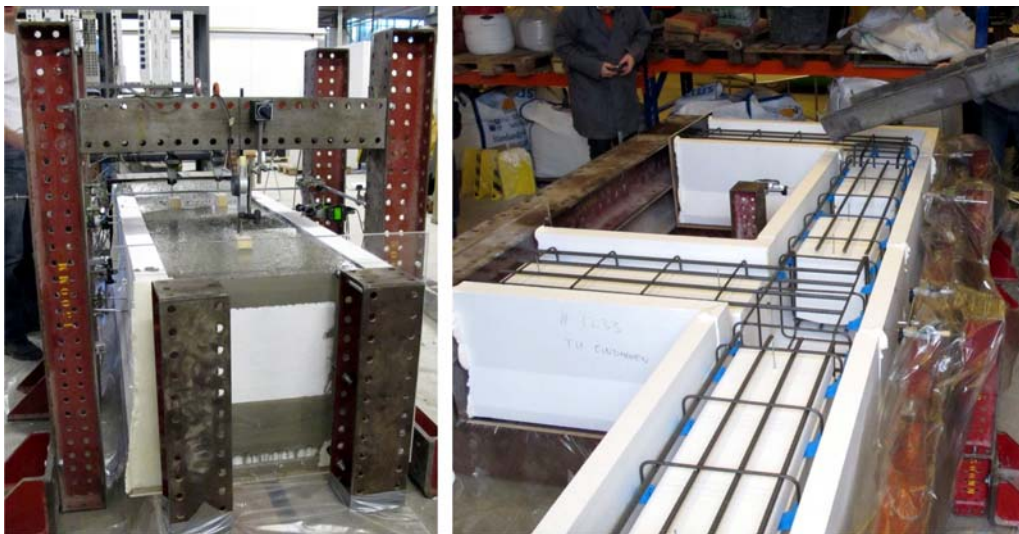
Fig. 4 Experimental casting using the new developed formwork system: straight segment of the foundation beam (left); casting of corner joint and T-joint (right)
